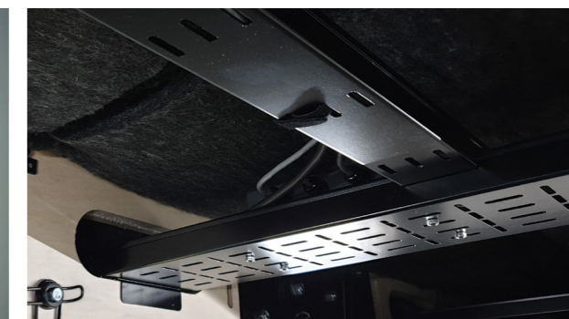
Cable-management within ceiling
