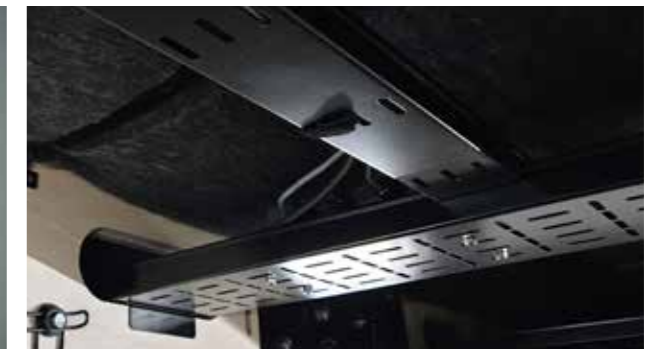
Cable-management within ceiling
